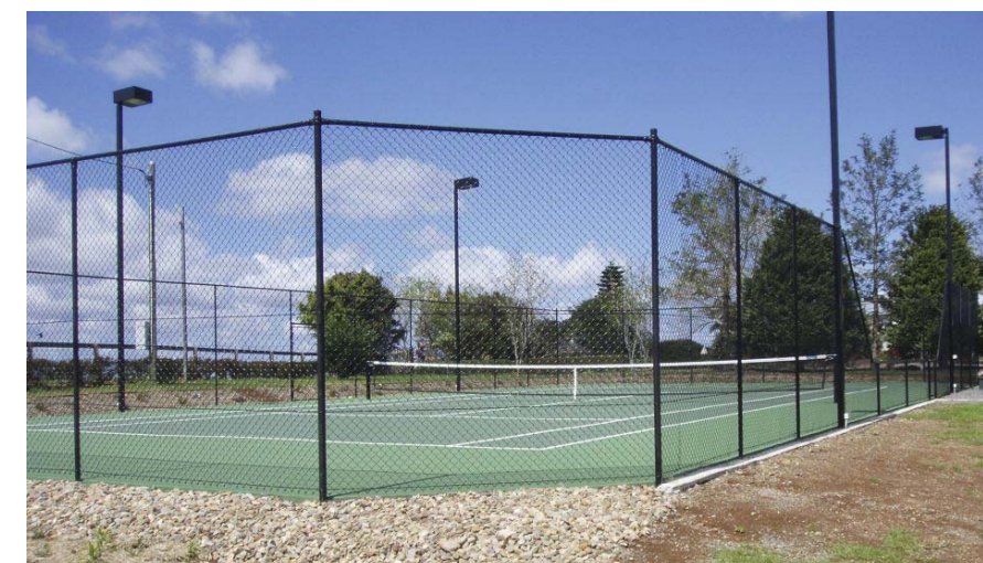
Tennis Court Fencing Black Vinyl Coated Chain Link - 12' high
