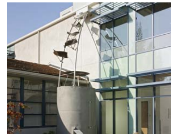
Rainwater is captured and used to flush toilets in Oakland.
