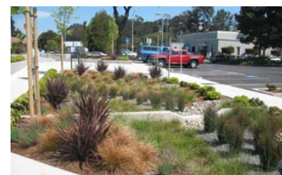
Rain garden collects and filters parking lot runoff in Brisbane.
